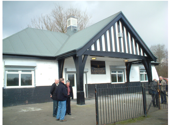
Renovated Boathouse Café 1.3.09.
