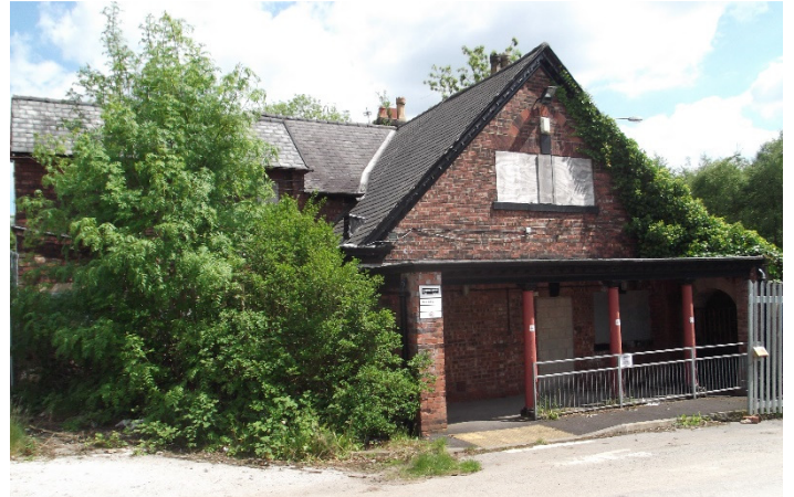
Photo 2, taken 3.6.2013: former hospital's Lodge Gatehouse.
