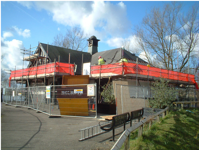
Boathouse exterior renovation work in progress 4.3.08.
